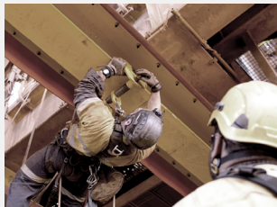
Difficulties to access bolt and nut to retighten
