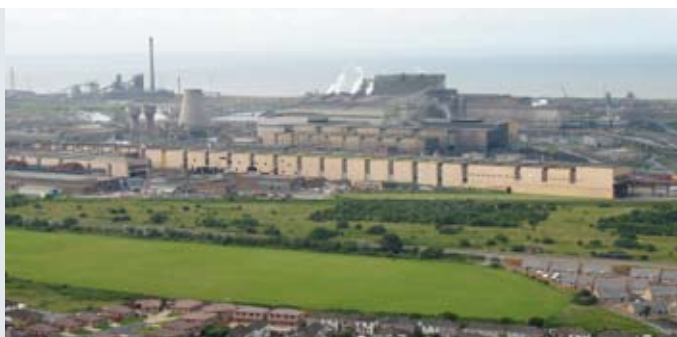
Corus integrated steelworks in Port Talbot, South Wales.
